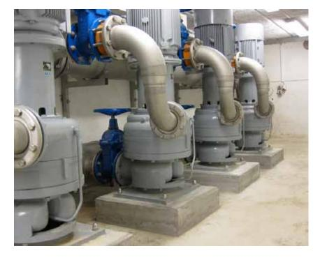
Pumps from Trium pump can be installed in a vertical position as shown from a supply in Roskilde. This is also possible onboard ships, where the removal space is limited.
